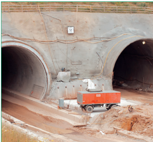
Fig. 1: Tunnel portal area
