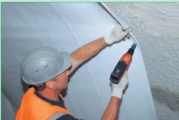
Fig. 25: Attaching Secutex® protection geotextile on the sealing carrier layer side wall
