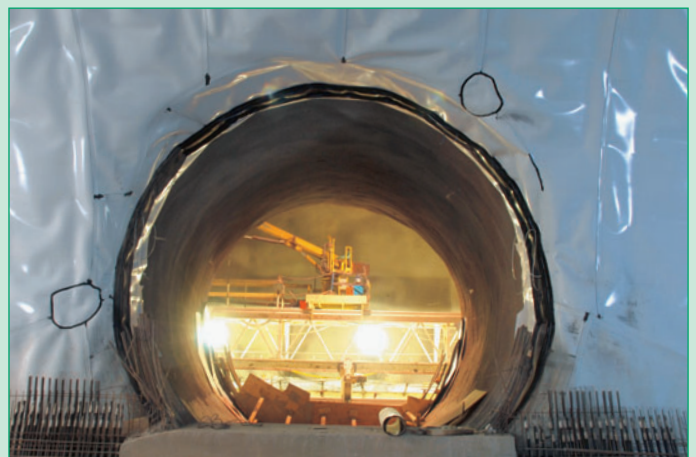
Fig. 21: 360° sealing in a connection tube
