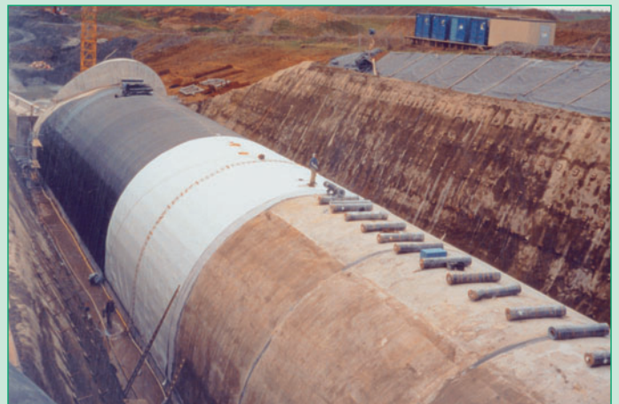
Fig. 23: Portal area with Carbofol® tunnel geomembrane
