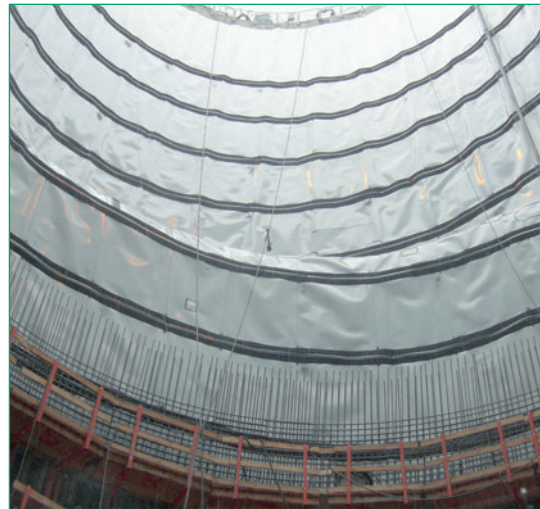
Fig. 35: Waterstop system in the shaft area
