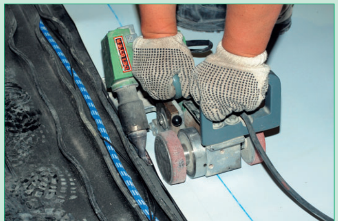
Fig. 34: Welding a waterstop to the Carbofol® tunnel geomembrane
