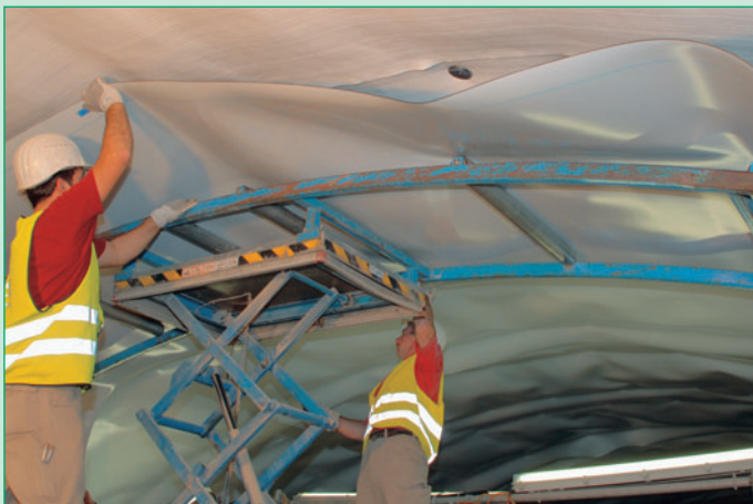
Fig. 29: Installing Carbofol® tunnel geomembrane in the arch
