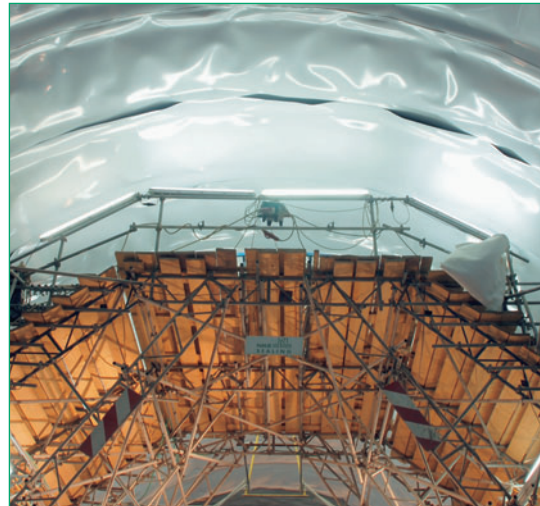
Fig. 31: Carbofol® tunnel geomembranes over an arch scaffold
