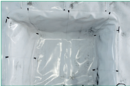
Fig. 32: Carbofol® tunnel geomembranes in the niche area
