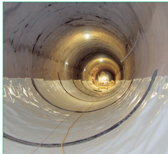
Fig. 3: Carbofol® tunnel geomembrane in the floor area
