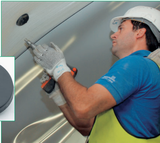
Fig. 27: Attaching the protection geotextiles using Carbofol® rondelles and a bolt gun
