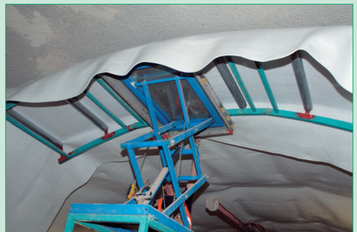
Fig. 26: Securing the Secutex® protection geotextile (arch area)
