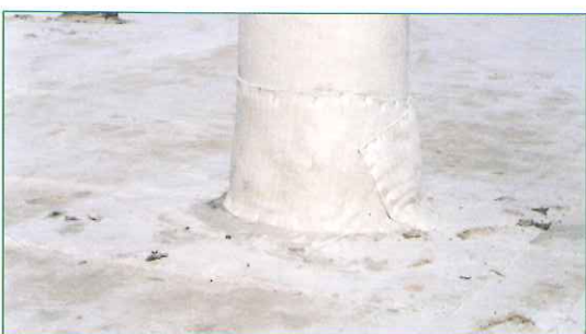
Sealed pipe penetration with BENTOFIX®
