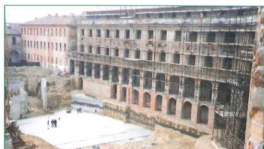
Waterproofing site with BENTOFIX®
