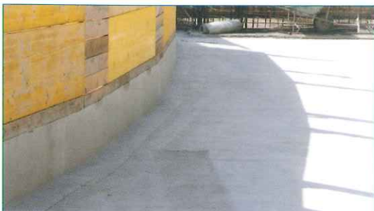
Vertical fixing of BENTOFIX®
