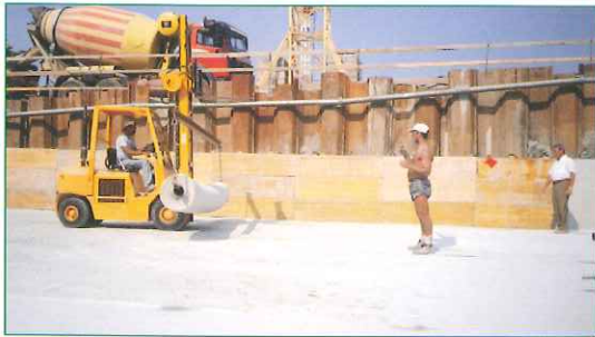
Transportation of a BENTOFIX® BFG 5000 maxi liner
