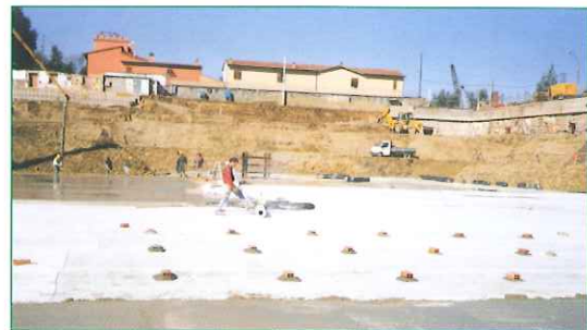
Unrolling of BENTOFIX® membrane on a base
