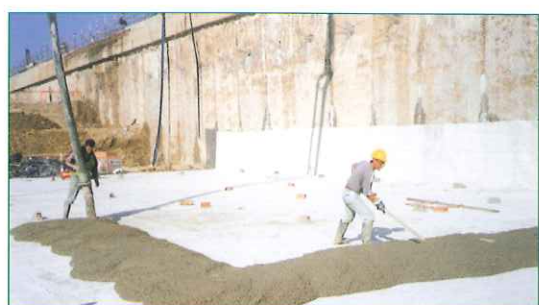
Pouring of concrete over BENTOFIX®
