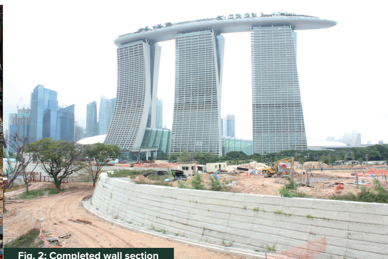
Fig. 2: Completed wall section
