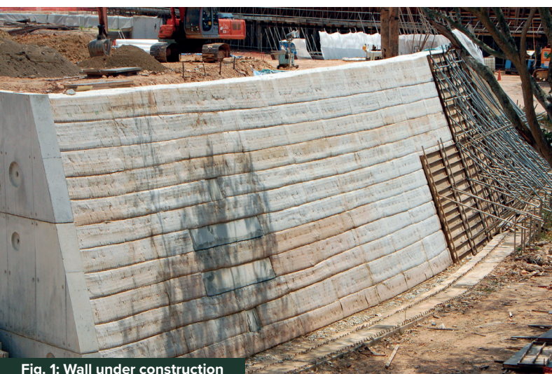
Fig. 1: Wall under construction
