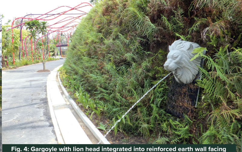
Fig. 4: Gargoyle with lion head integrated into reinforced earth wall facing
