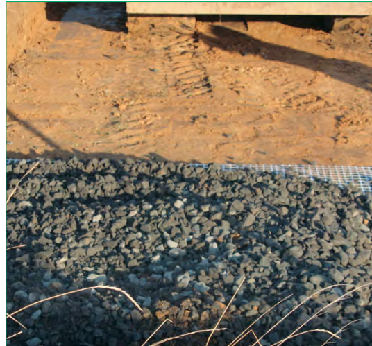
Fig. 17 Placement of base course gravel over the Secugrid® section
