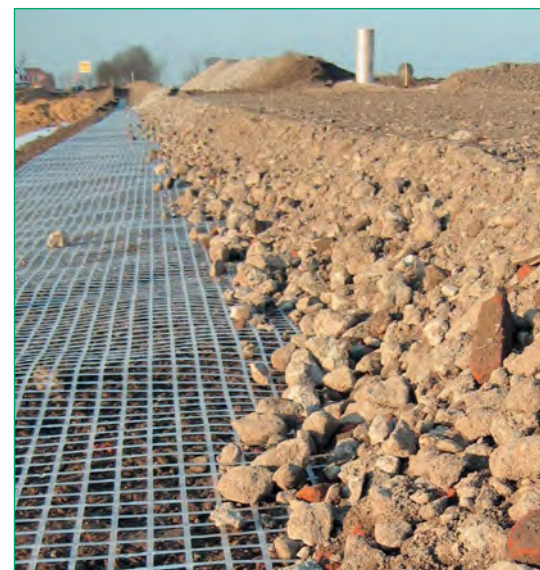
Fig. 19 Crushed base course material over Secugrid® for base stabilisation in access roads
