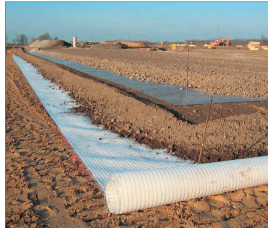
Fig. 8 Base course reinforcement on a very soft subsoil with Combigrd® (bottom) and Secugrid®
