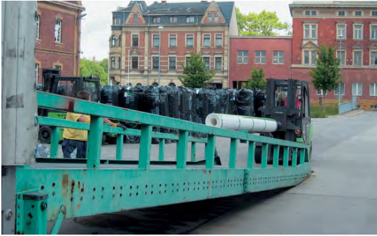
Loading of Secugrid®
